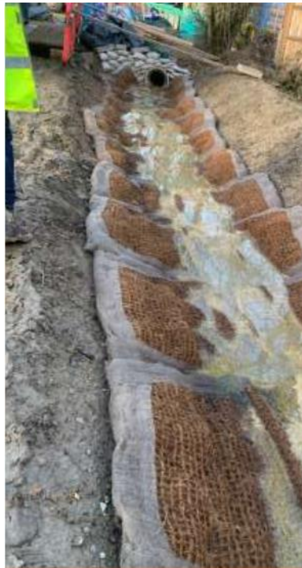
Trench with flocculant matting
